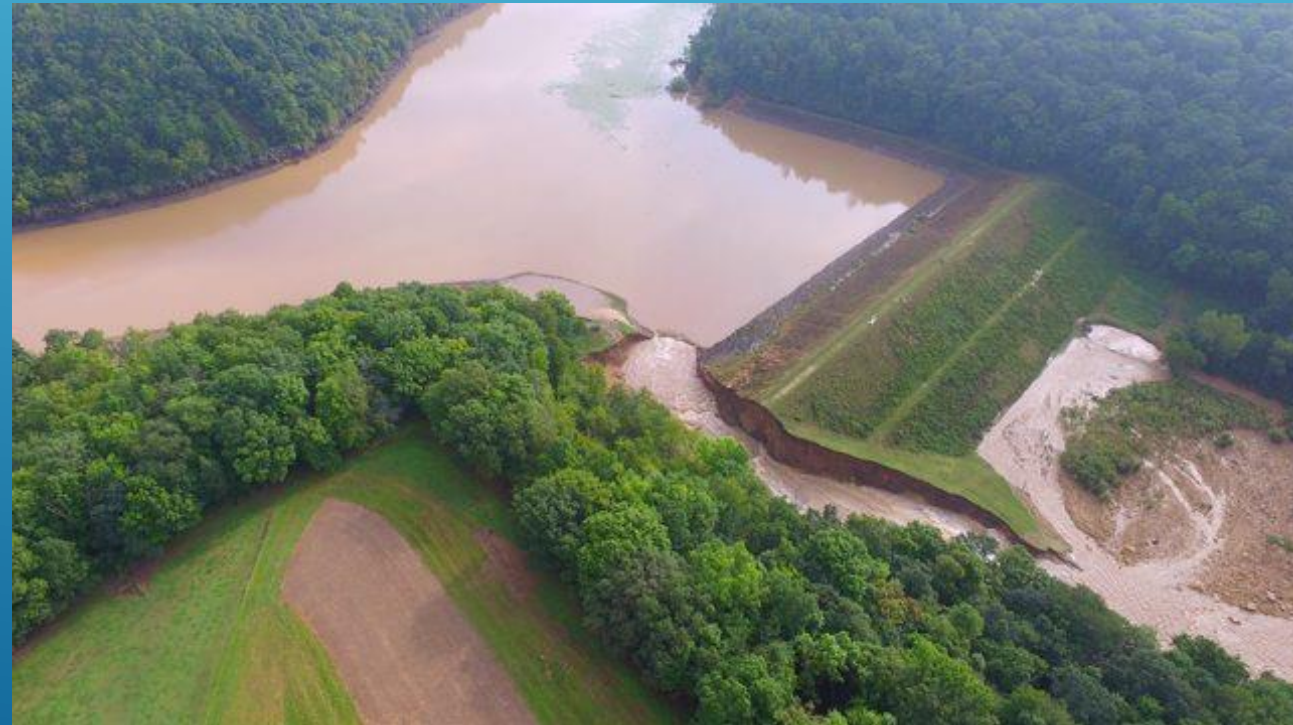
Jersey Valley – Dam Breach – (Kickapoo)
