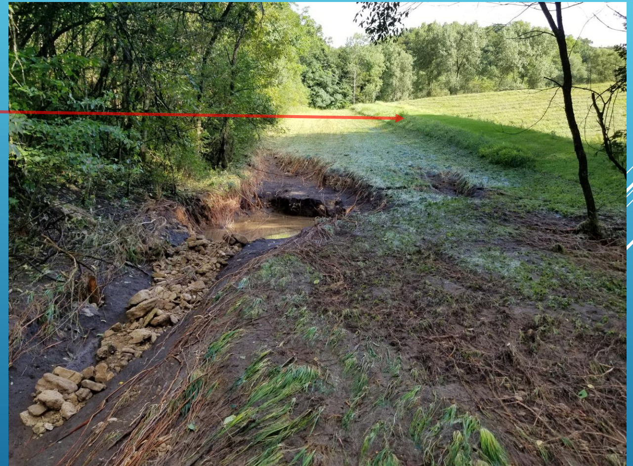
Emergency/Auxiliary Spillway Repair
