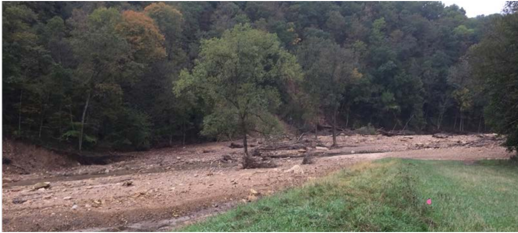
Photo 42 View downstream of dam of outwash from left abutment. (CC 21)
