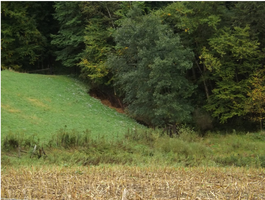
Photo 31 Erosion in left groin. (WFK 3)
