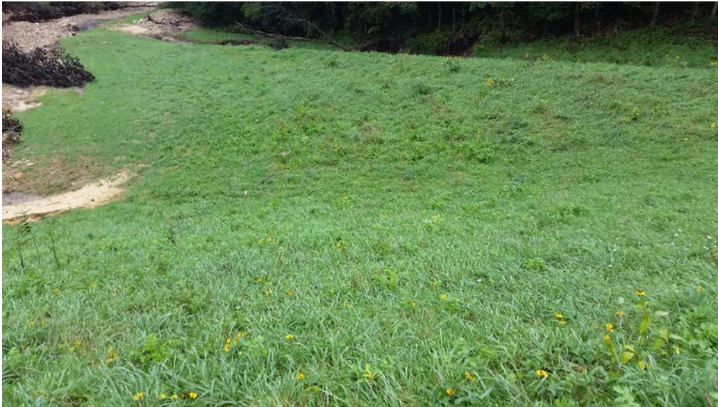
Photo 65 View of right groin from top of dam. (CC 23)
