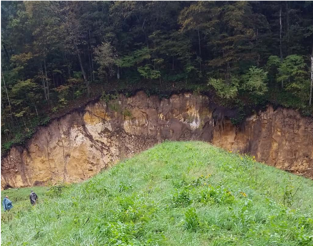
Photo 69 View of exposed bedrock in left abutment – breach channel. (CC 23)
