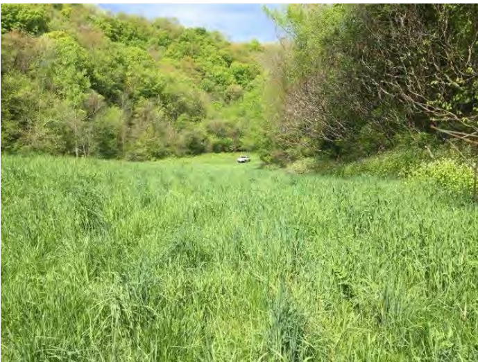
0036105181611 Auxiliary spillway crest looking downstream
