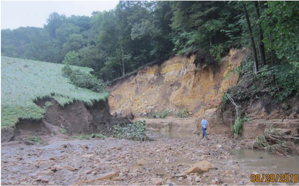
Photo 67 View of breach channel from downstream of dam. (CC 23)
