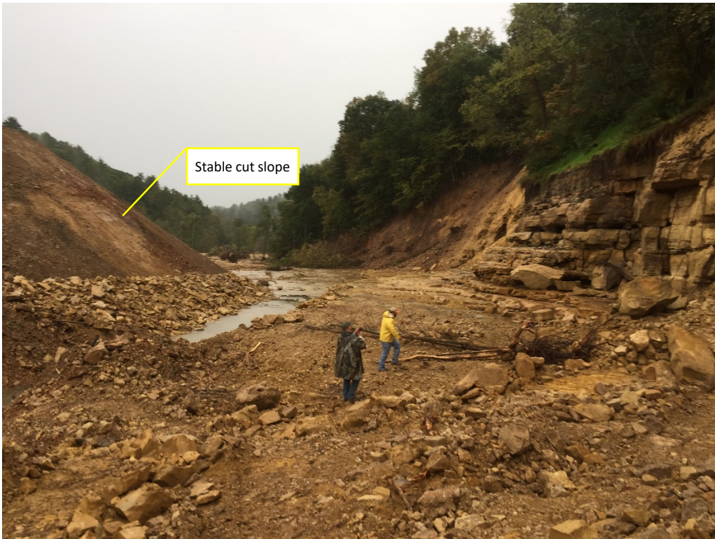
Photo 2 View of Breach Channel from Upstream (WFK 1)
