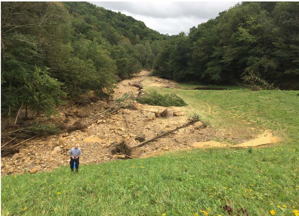
Photo 70 View of debris in breach inundation area downstream of dam. (CC 23)
