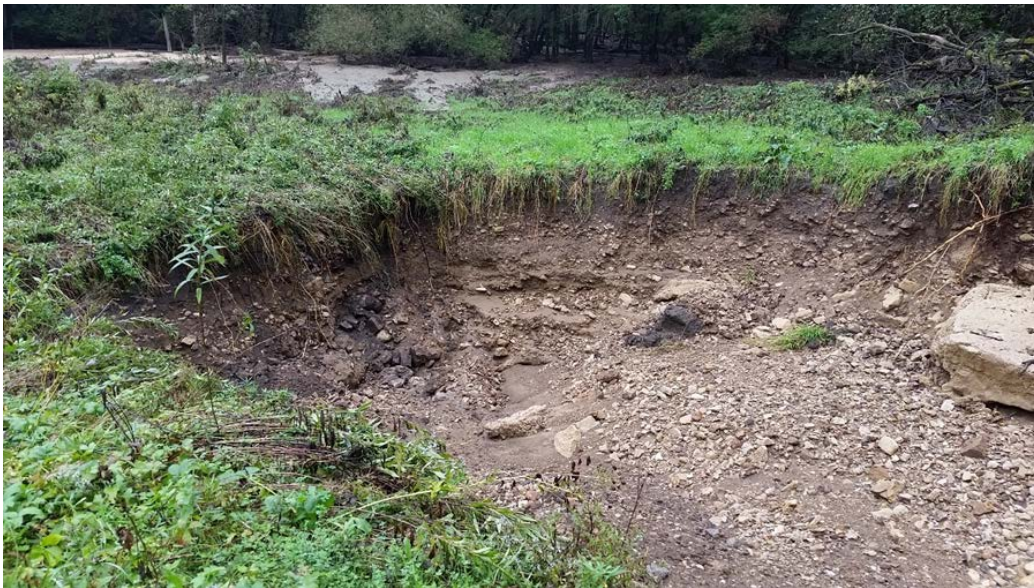
Photo 66 Head cut into upstream sediment pool due to breach of dam. (CC 23)
