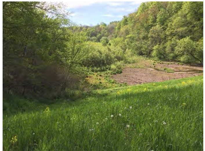
0036305181612 Auxiliary spillway crest looking upstream
