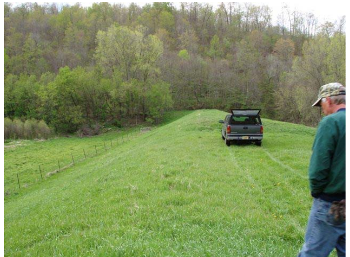
0035804262012_19 Auxiliary Spillway Inlet Channel
