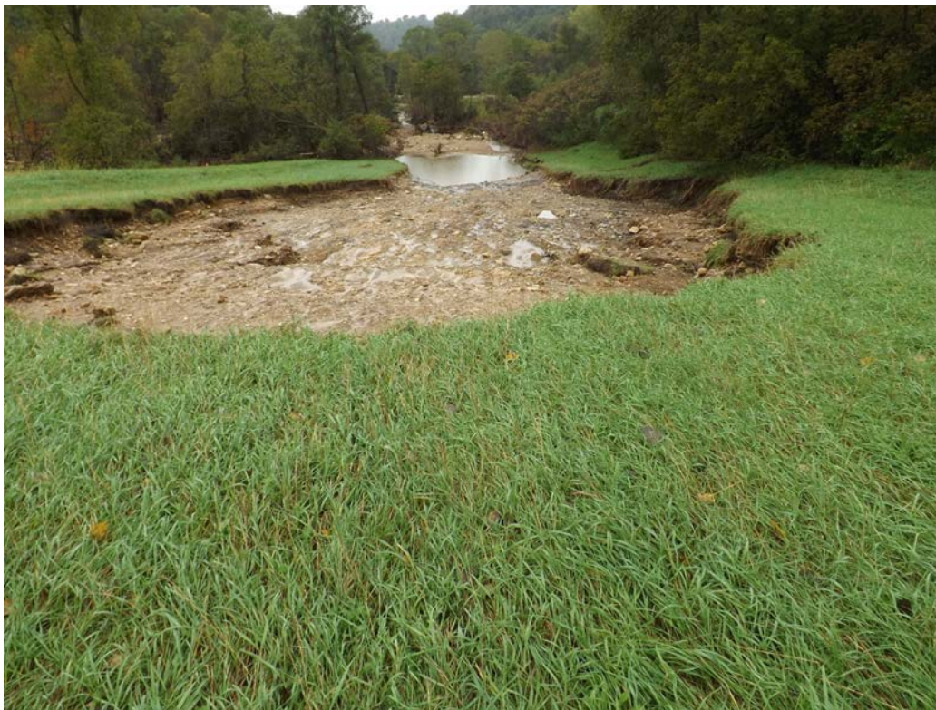
Photo 45 View of auxiliary spillway exit channel from level section. (CC 29)
