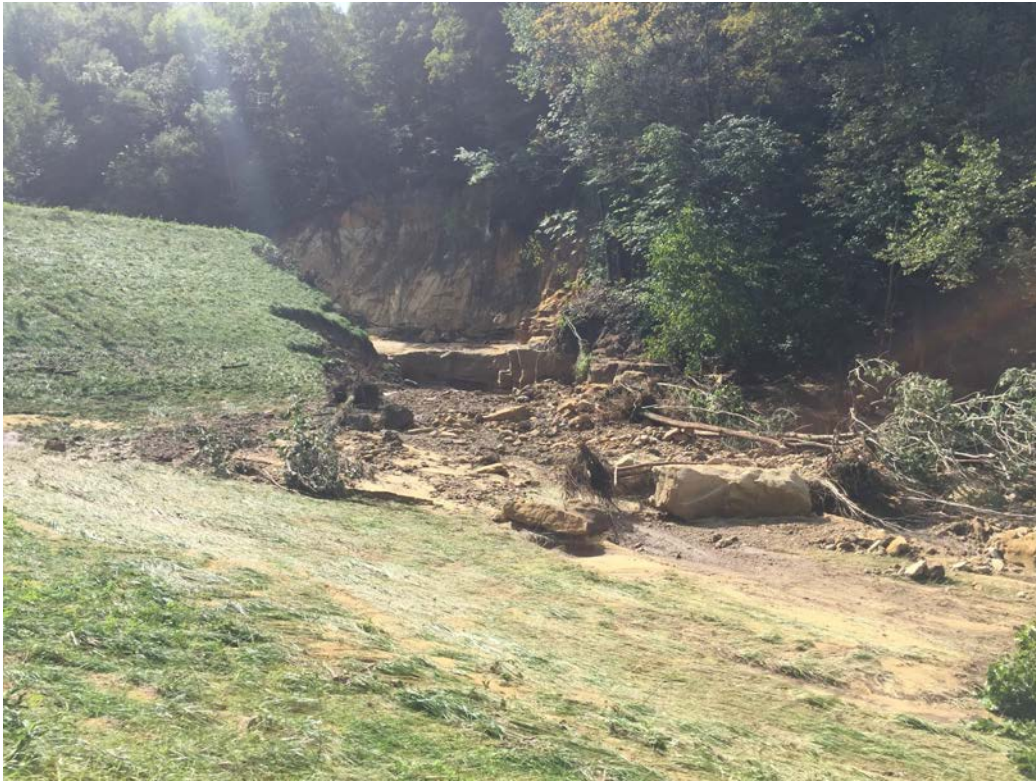
Photo 71 View of head cut into bedrock of breach channel. (CC 23)
