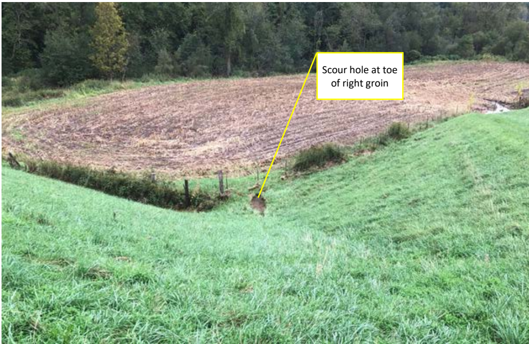
Photo 30 View of right groin from top of dam. (WFK 3)
