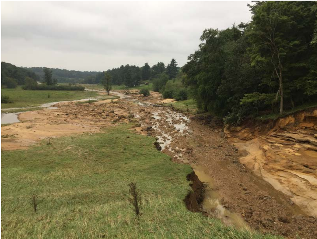
Photo 24 View of breach inundation area from top of dam. (WFK MLSNA)
