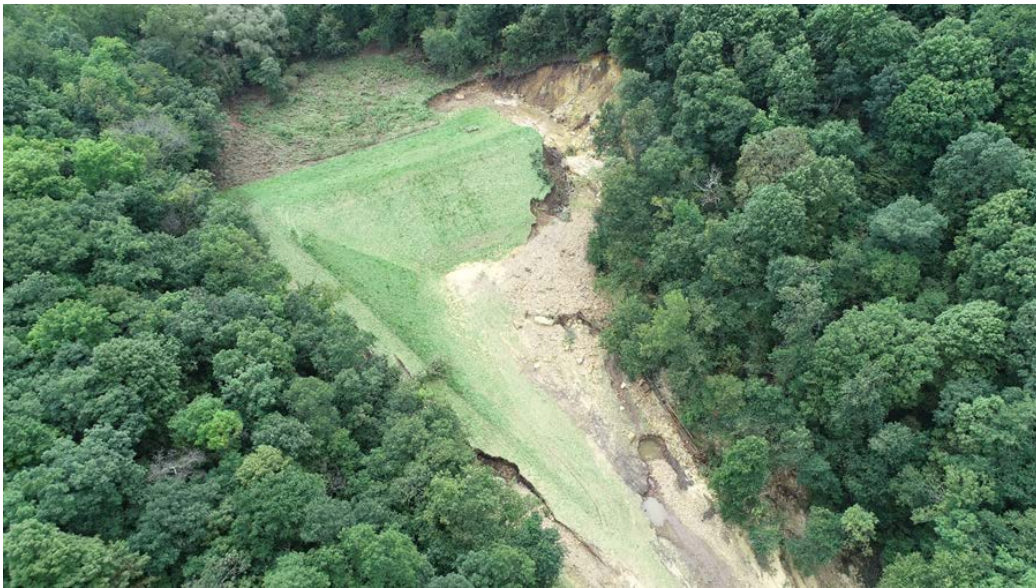
Photo 55 Aerial view of structure site. (CC 23)
