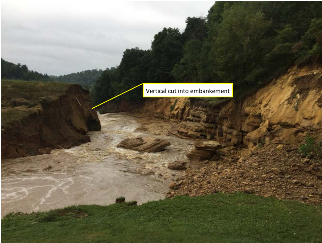
Photo 1 View of Breach Channel from Upstream (WFK 1)
