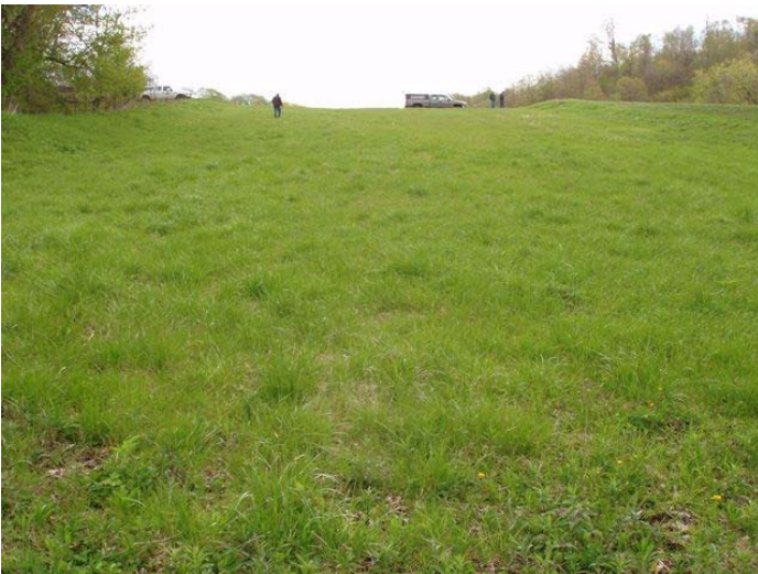
0035804262012_01 Auxiliary Spillway Exit Channel
