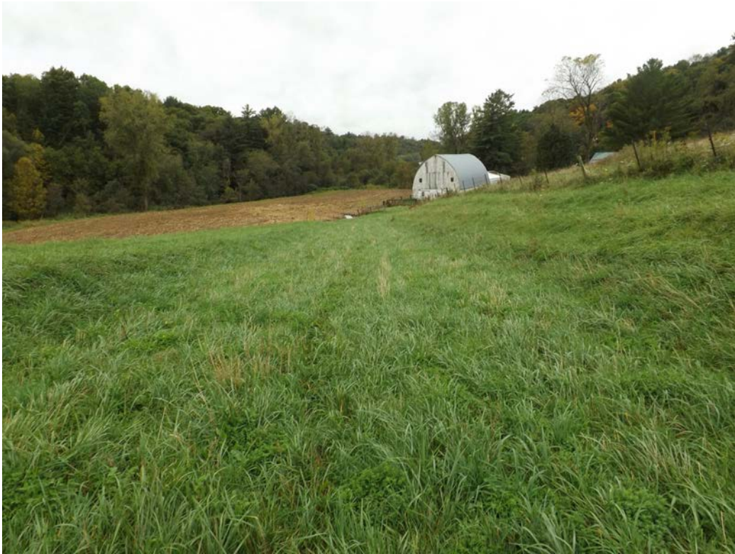
Photo 28 Exit channel of auxiliary spillway. (WFK 3)
