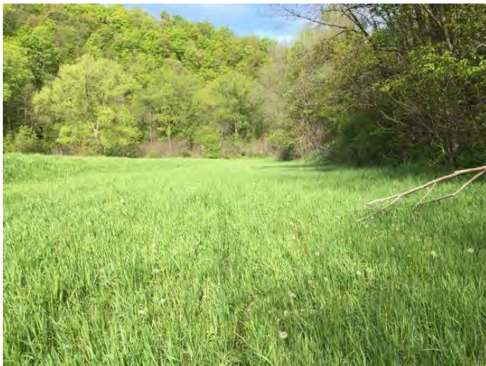
0036305181611 Auxiliary spillway crest looking downstream
