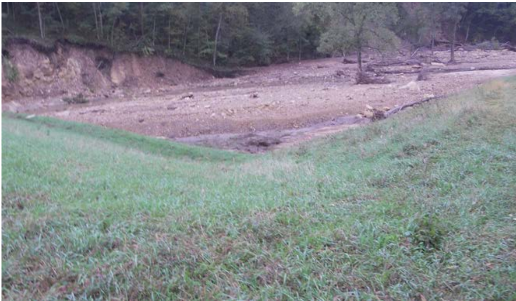
Photo 41 View of right downstream groin from top of dam. (CC 21)
