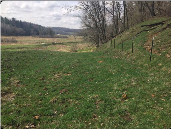
00393050318_07 Auxiliary spillway looking downstream
