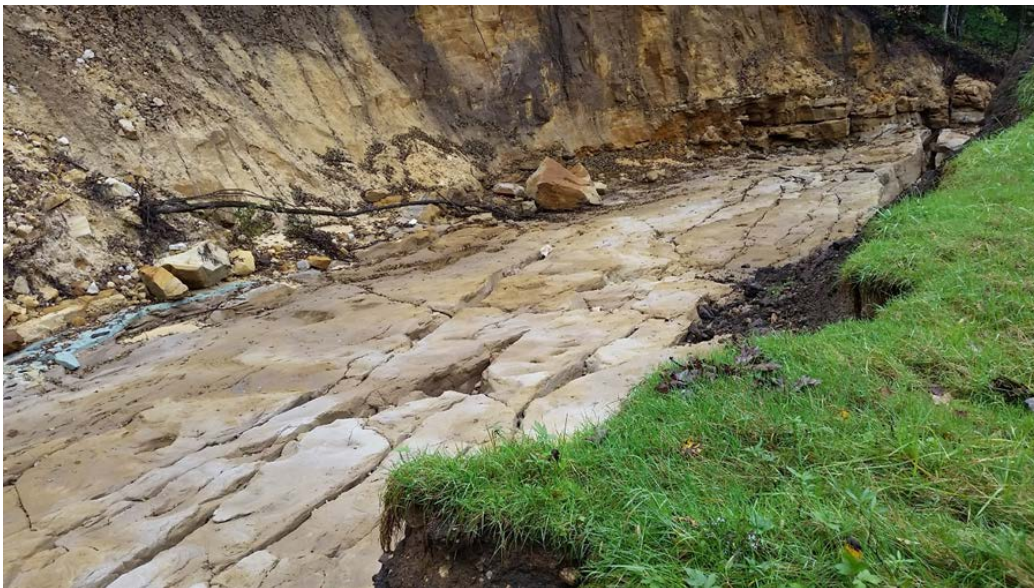
Photo 68 View of breach channel from upstream toe of dam. (CC 23)
