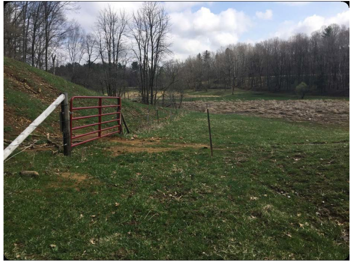
00393050318_08 Auxiliary spillway looking upstream
