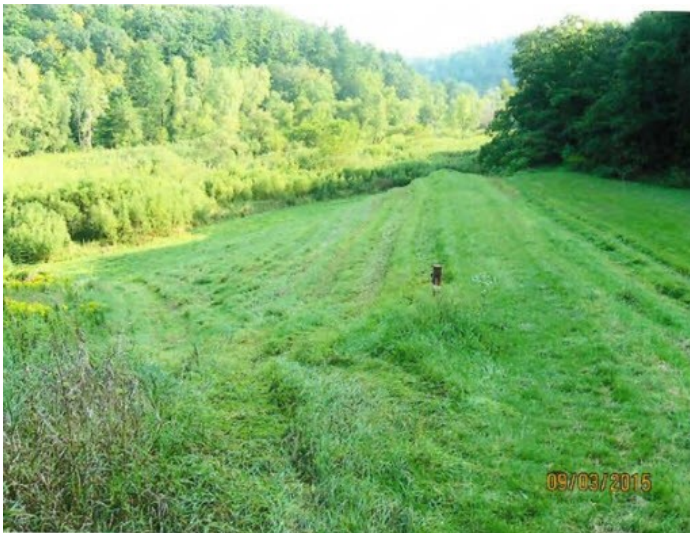
Auxiliary Spillway Looking Downstream
